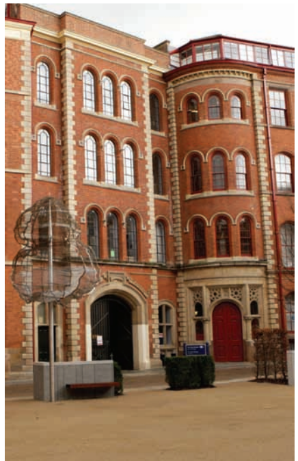
The rear of the Adams Building today
